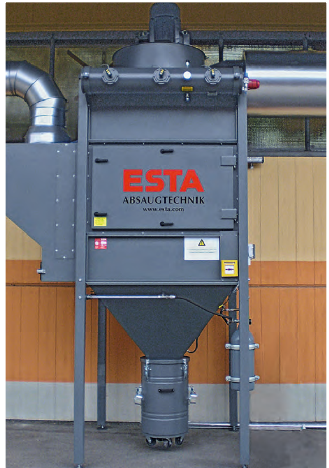
DUSTMAC F-96 central welding fume filter system with integrated ABC powder extinguishing system
