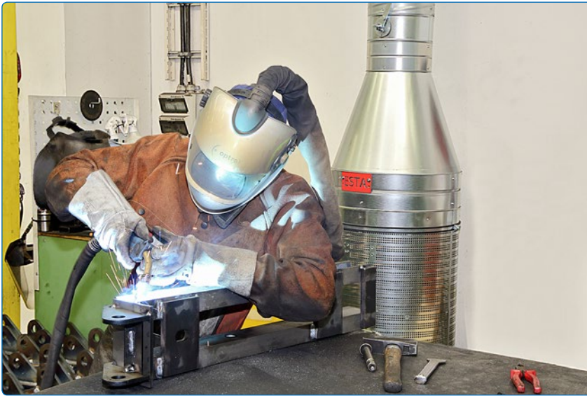
Displacement diffusers are installed in all welding workstations.
