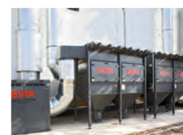
Pipe system as a supply line for central extraction system
