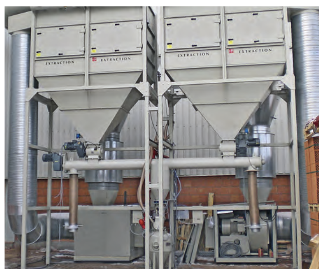
Central extraction system with two rotary valves for the continuous discharge of brick dust
