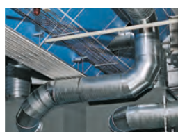
Connecting pipe between fan and filter system
