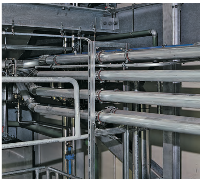
Steel pipe system of a central extraction system in the tobacco industry
