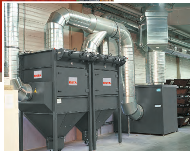
Post-filters installed on the DUSTMAC F-288 central extraction system
