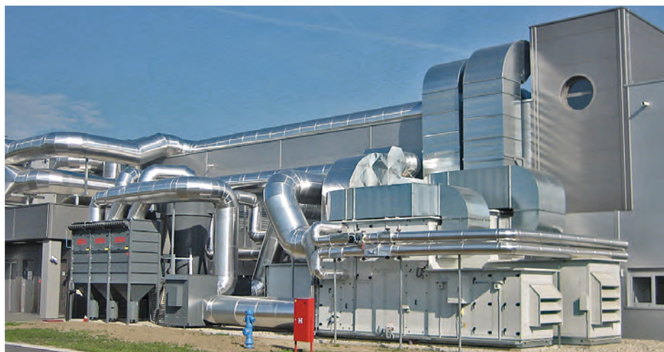
Central extraction system with spiral seam pipes system in the shoe industry
