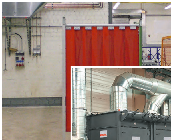
Post-filters on a filter system in a metal working shop
