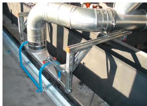
Slotted vacuum channel for the extraction of metal chippings
