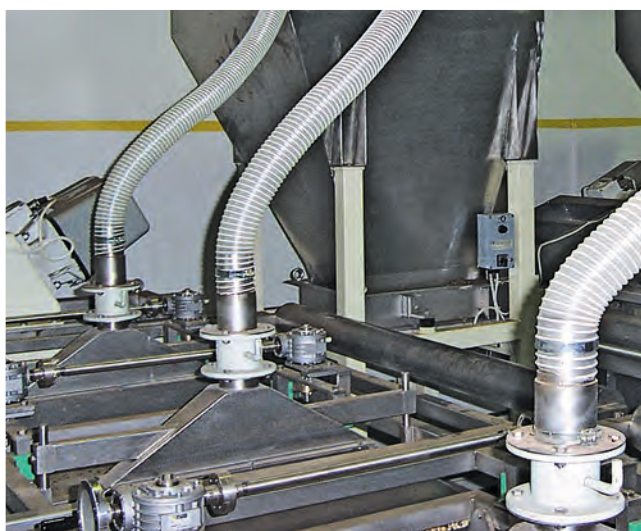
PU hoses for connecting the extraction hoods to the pipe system in a metalworking shop
