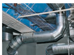
Connecting pipe between fan and filter system
