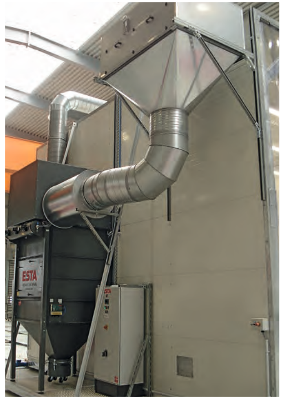
Modular ESTA extraction system DUSTMAC F-144 with post-filters for the extraction of GFK sanding dust
