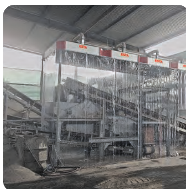
Extraction hoods over conveyor belts
