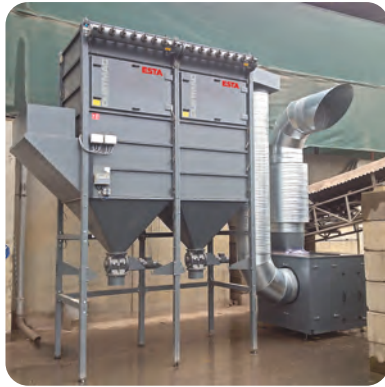
Extraction unit DUSTMAC S-66 and medium-pressure fan
