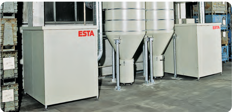
High pressure fans combined with ESTA filter cyclones
